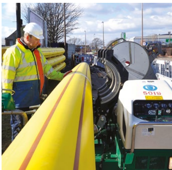
Large Diameter Main Laying
